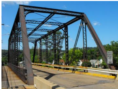
Metal 7 Panel Pin-Connected Pratt Through Truss, Fixed Length: 109 ft. Main Span: 105 ft. Roadway: 19 ft. Main Spans: one Built 1886 By: Morse Bridge Company of Youngstown, Ohio
