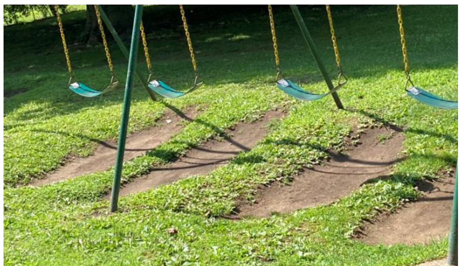
No safety surface under swings
